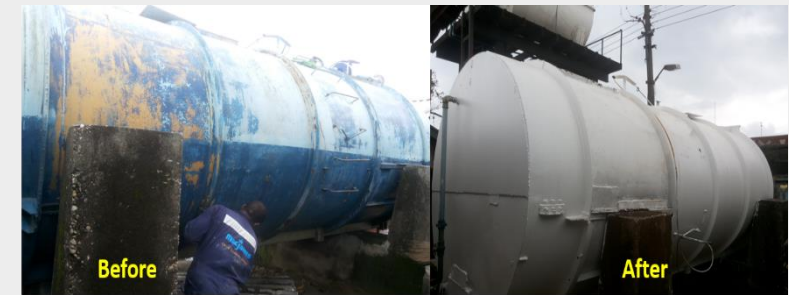
Surface Cleaning and Anti-Corrosion Coating of SeWa Raw Water Storage Tank
